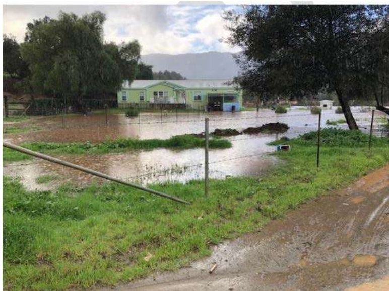
Figure 9. Flooding at a Pala home, February 2019
